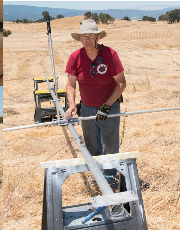
Below left, Rebar, N6DB waiting for the next tower tube
