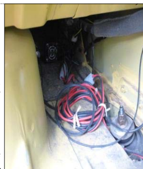
Fig 3: Main radio unit in trunk cavity
