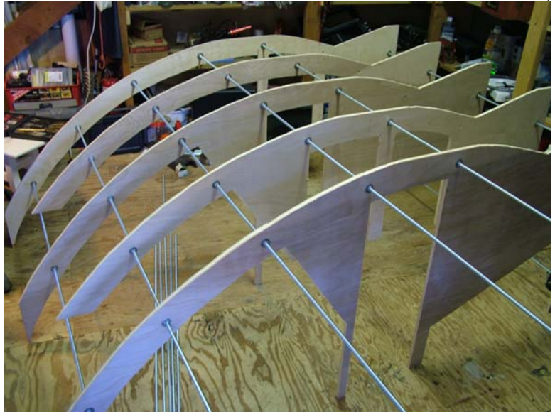
Photo 11, radio deck, under construction
